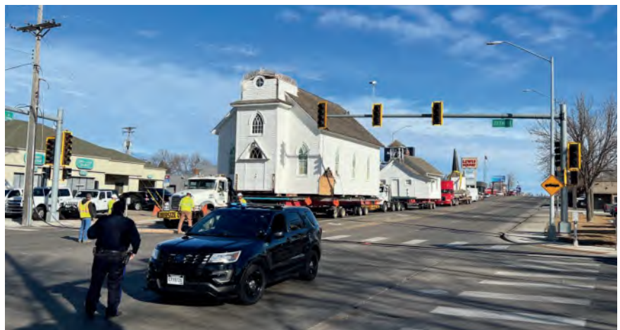
Two buildings are moved from Augustana University campus due to expansion of the college athletics complexes.
