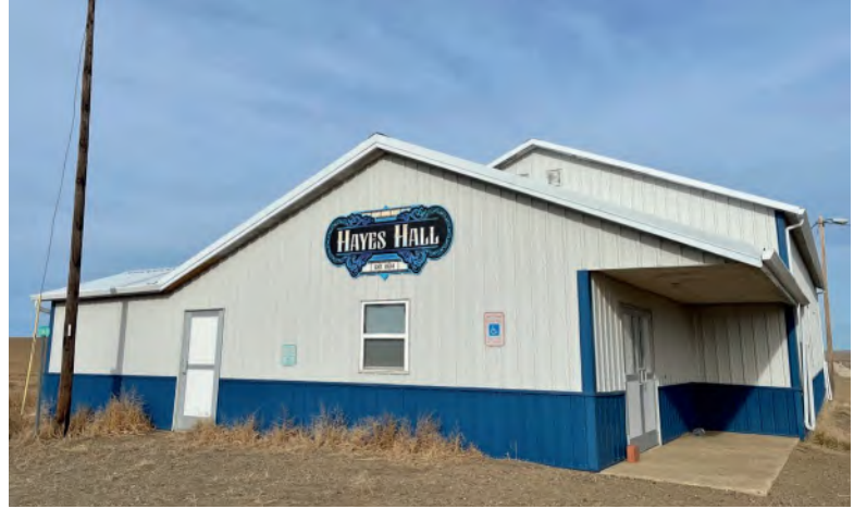
For a few nights every year, Hayes Hall gets packed to standing-room only. West Central Electric Cooperative provides the hall's electrical power and is an annual sponsor of the Hayes play.
